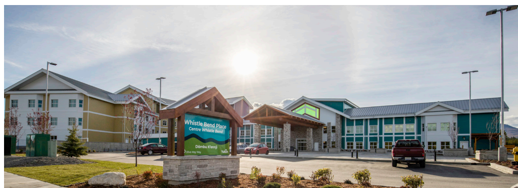
PHOTO CREDIT: PCL Constructors Westcoast INC.
